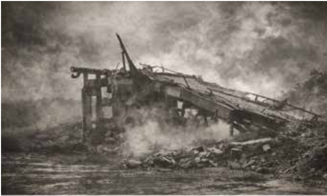
Civil engineers ensured destruction was strategic, not chaotic.
