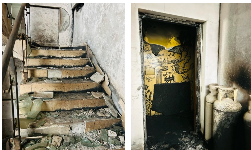
Figure 07: Damaged staircase due to excessive heat (L) and damage doors due to fire (R)
