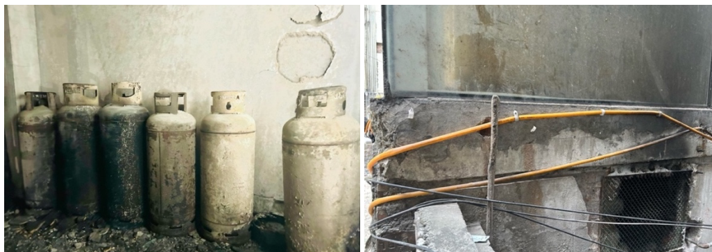
Figure 06: LPG cylinders stored at the staircase (Left) and gas line connection using flexible plastic pipeline (Right)
